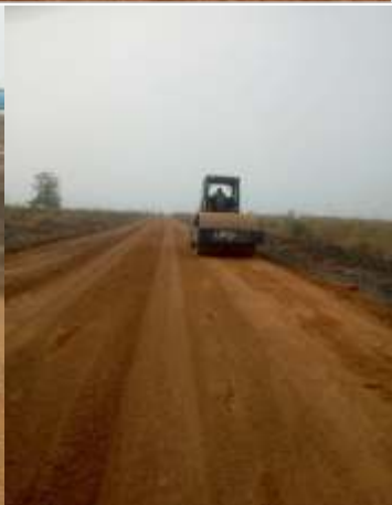
Grading of Access Road in Plateau State.
